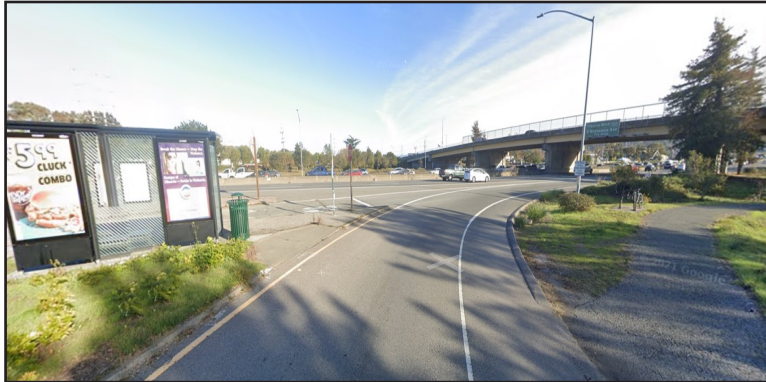
Existing pedestrian route to SB bus stop requires unprotected crossing of SB 101 loop onramp
