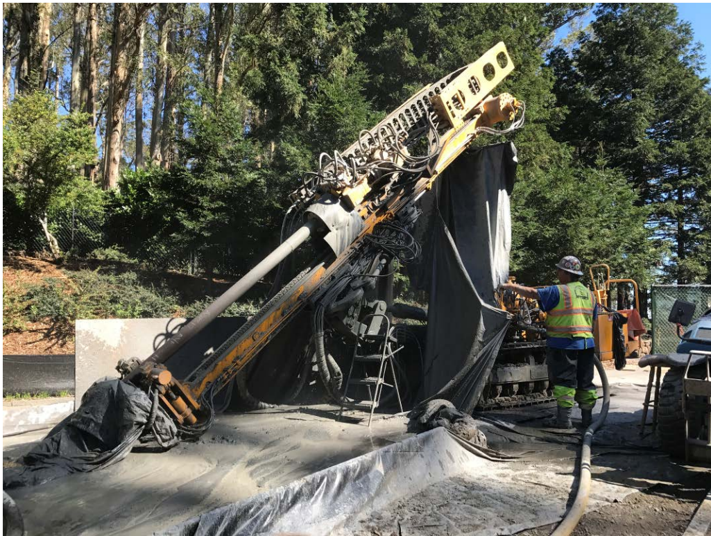
Photo 4. Klemm drill being utilized for the borehole drilling of BH-3 at the Chapman Site location.
