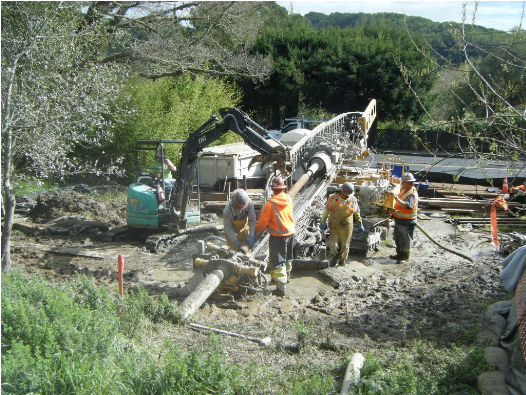
Photo 3. Klemm drill being utilized for the borehole drilling of BH-2 at the Underhill Site location.
