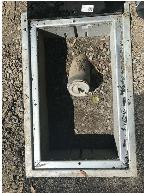
Photo 5. Typical concrete Christy box installation to seal each borehole following the investigation.
